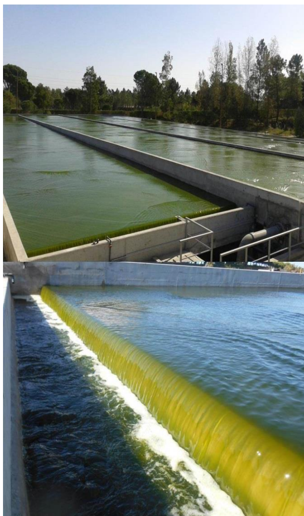
BIOFAT Pataias Pilot Plant Cascade Raceway – 2 x 1500 m 2 – Designed and built by A4F. (BIOFAT FP7 project)
