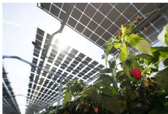
Figure 6.3 Raspberry farm with PV arrays as protective roof. Babberich, the Netherlands.
