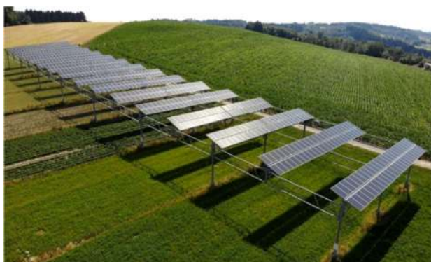
Figure 6.4 Configuration of PV arrays in APV Research Plant in Heggelbach, Germany.
