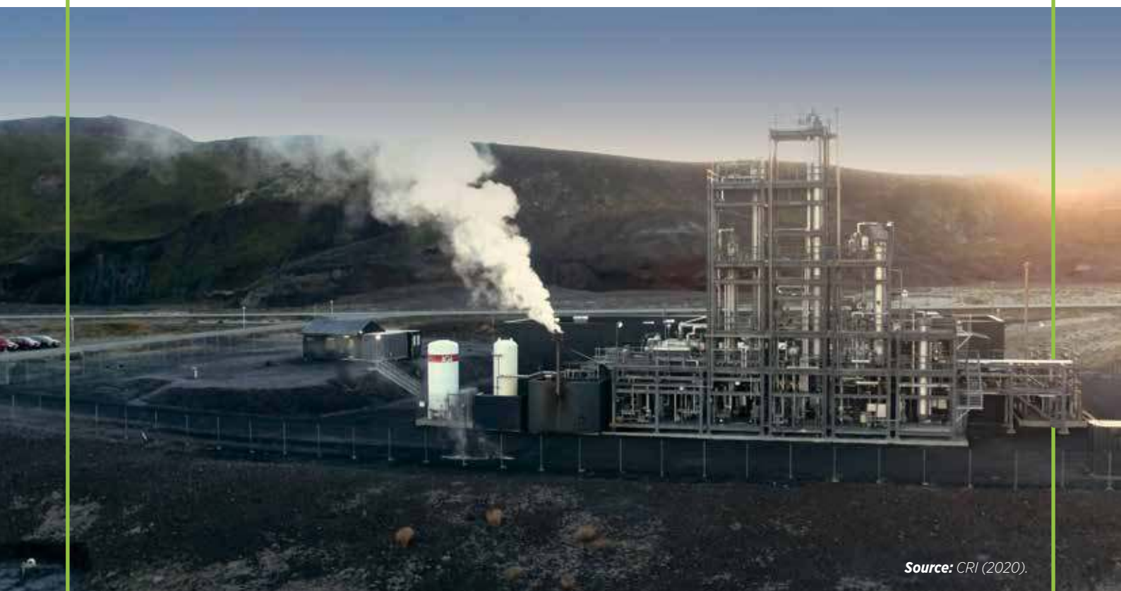
Figure 26. The “George Olah Renewable CO 2 -to-Methanol Plant” of CRI in Iceland
