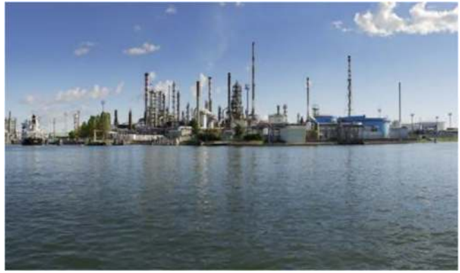
Photo 14 ENI's Green Refinery plant in Venice
