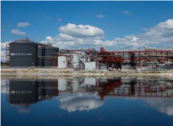
Photo 15 UPM's Lappeenranta biorefinery plant
