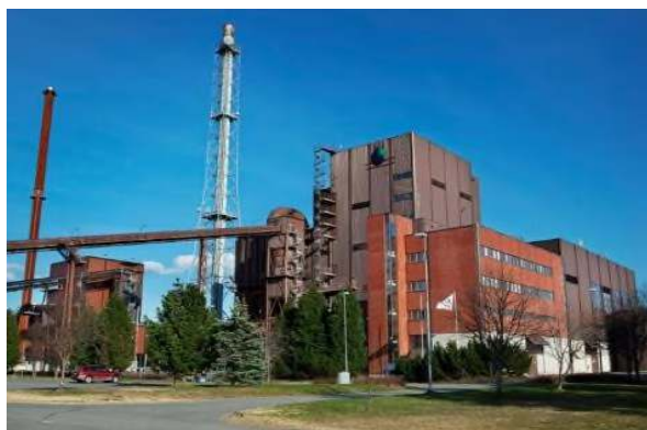
Photo 9 Fortum's Joensuu plant in Finland
